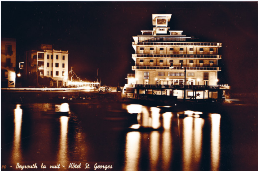
Top Saint Georges Hotel, Beirut Postcard, 9×14 cm Publisher: Photo Sport, Circa 1934-40 The Fouad Debbas Collection / Surssock Museum
